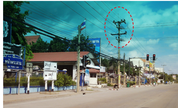
Figure 4: Insulator installation in pollution area.
