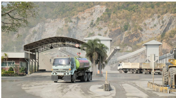
Figure 3: Cement dust particles in factory area.
