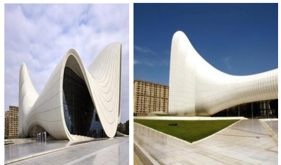
Figure 17: To protect intricate building structures from corrosion [70].
