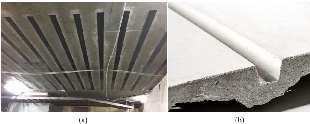
Figure 12: In the seismic repair of beam-column joints and production of composite concrete [42].
