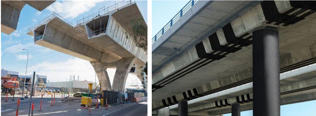
Figure 10: In the repair of the collapsed bridge [42].
