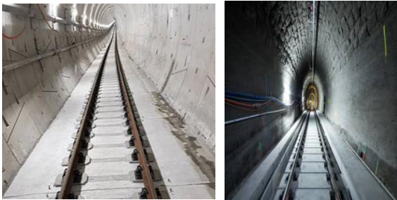
Figure 14: In repair and renovation of tunnels [73].
