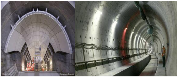
Figure 13: In the fabrication of materials for tunnel construction [73].
