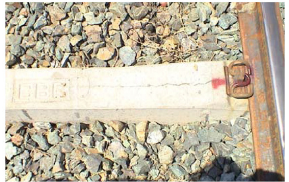
Figure 4: Crack in concrete sleeper. Adapted with permission [38].
